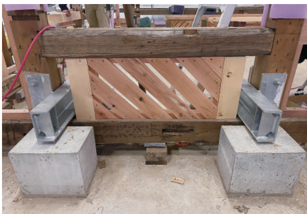
5 床下鉄骨材と斜め木摺壁
